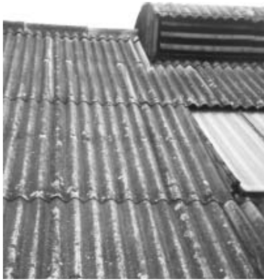
10b Asbestos cement roof (weathered exterior).
