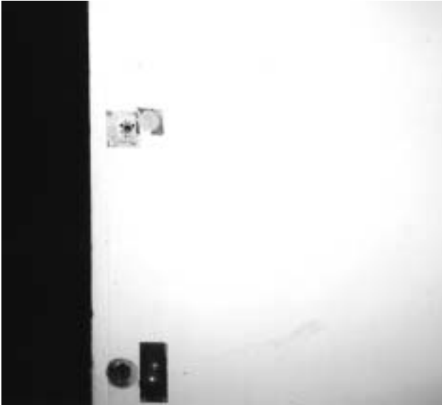
5g Painted AIB facing to a fire door with some damage around the door furniture.
