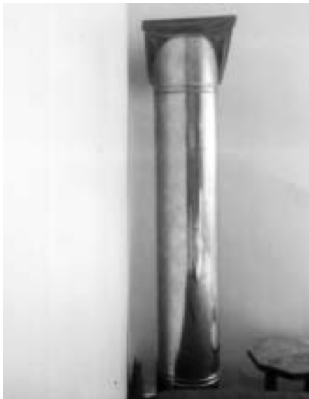
16a Metal-clad asbestos flue pipe.
