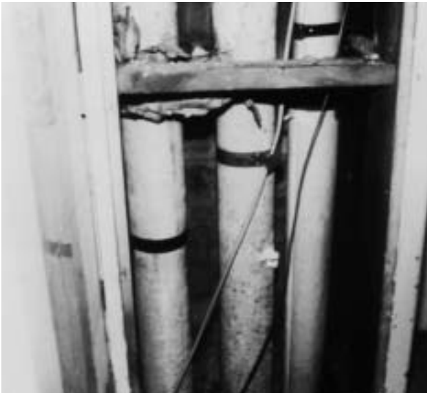
3c Asbestos pipe lagging in a service riser, with calico wrapping and straps.
