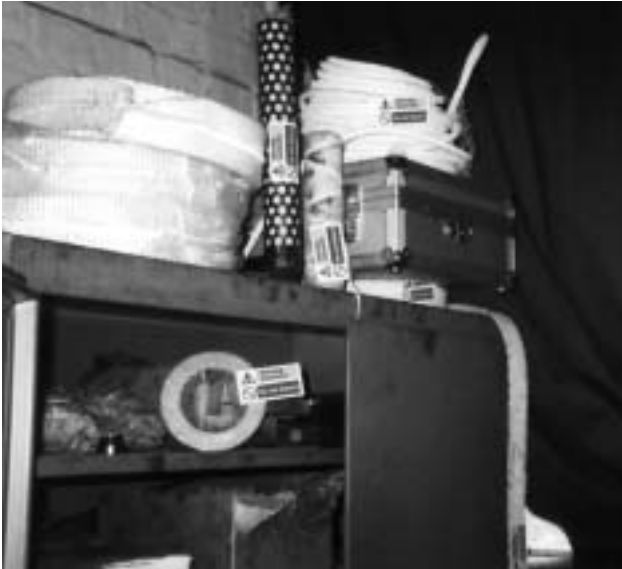
9a Asbestos tape, string, rope and gasket in a maintenance repair cabinet (note also the shiny vitreous appearance of a non-asbestos MMMF replacement tape to the left).
